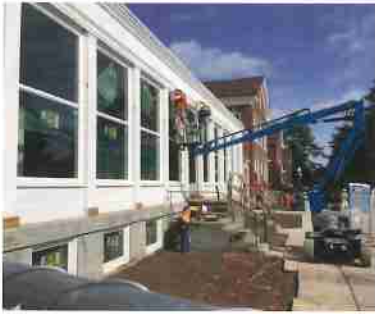
Construction of Mercy Magnuson Place is expected to finish in July 2019.
